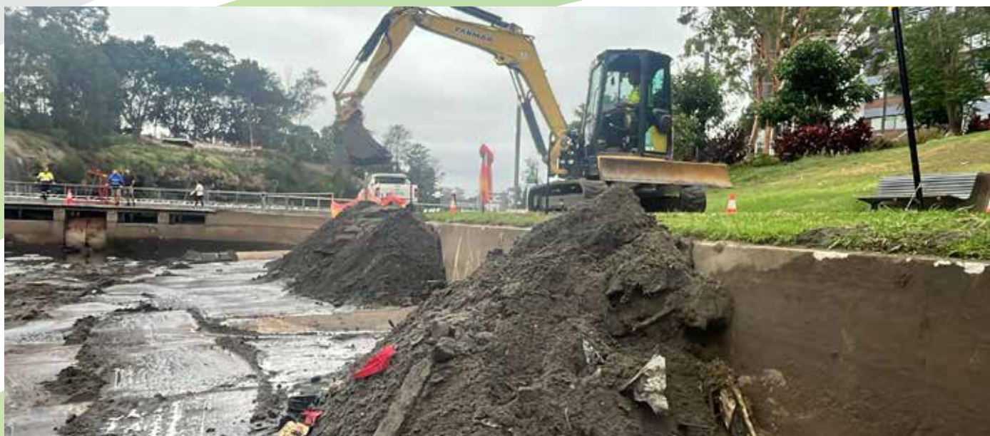
a) Picture Above Using Excavator to collect debris and sediment.
