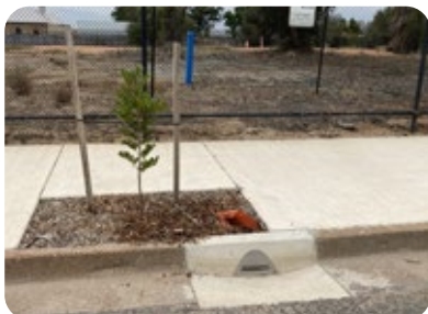
Space Down Under, in collaboration with Port Pirie Regional Council, as recently installed 130 Kerb Space Inlet Systems for passive irrigation of street trees.
