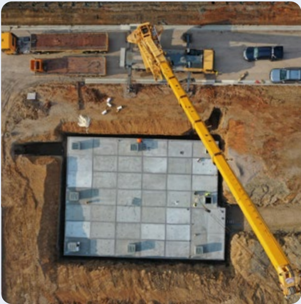
Four MegaVault tanks were installed at the site.
