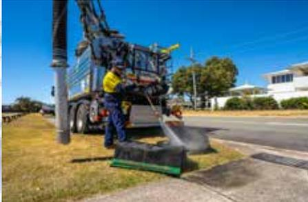
It is important that, prior to commencing a clean, you confirm all plant and equipment is available and operational with service records and pre-start checklists available. It is also recommended that weather conditions for the day of the proposed clean be confirmed as the clean can only be completed in dry weather conditions.
