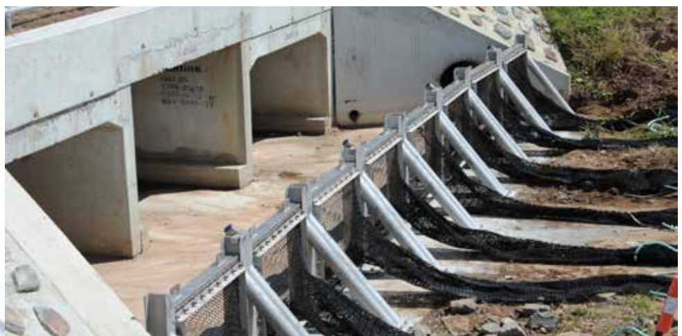
Site 4 Retained Pollutant Composition and volume (3rd March 2013 - 29th april 2014)
