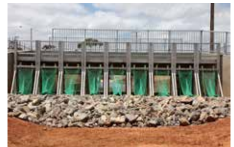
Figure 2 – Ecosol™ Nine module Trash Rack installation.
